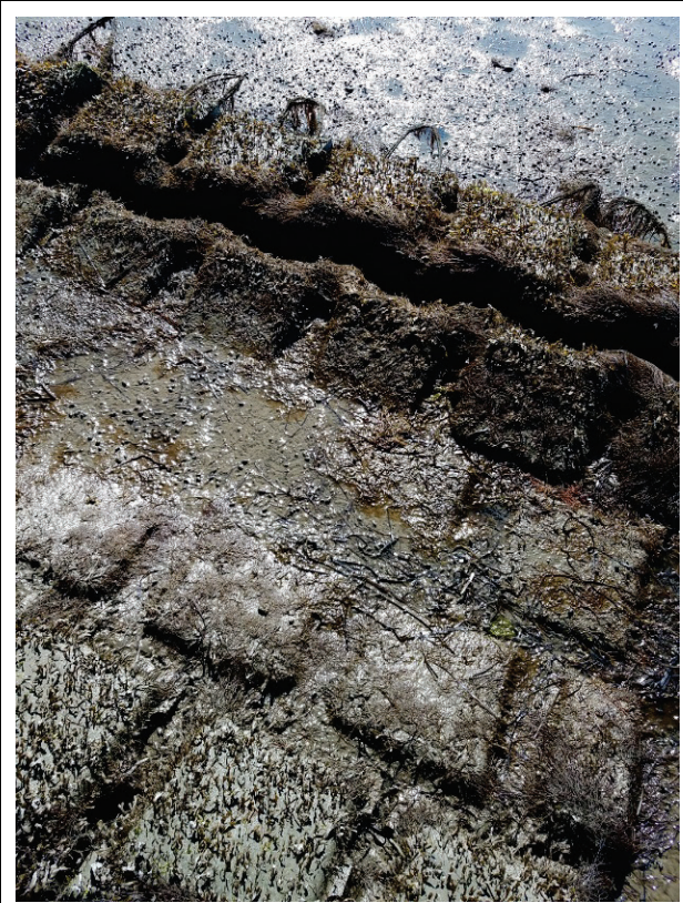
Figure 4. SRP concrete mattresses, with sediment, algae and snails on blocks, September 21, 2020.
